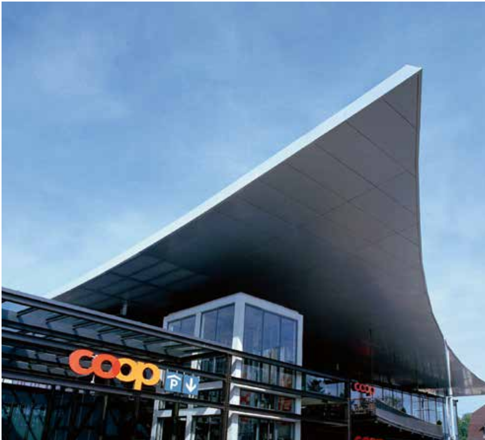
Stable – large, self-supporting roof with ALUCORE® cladding
